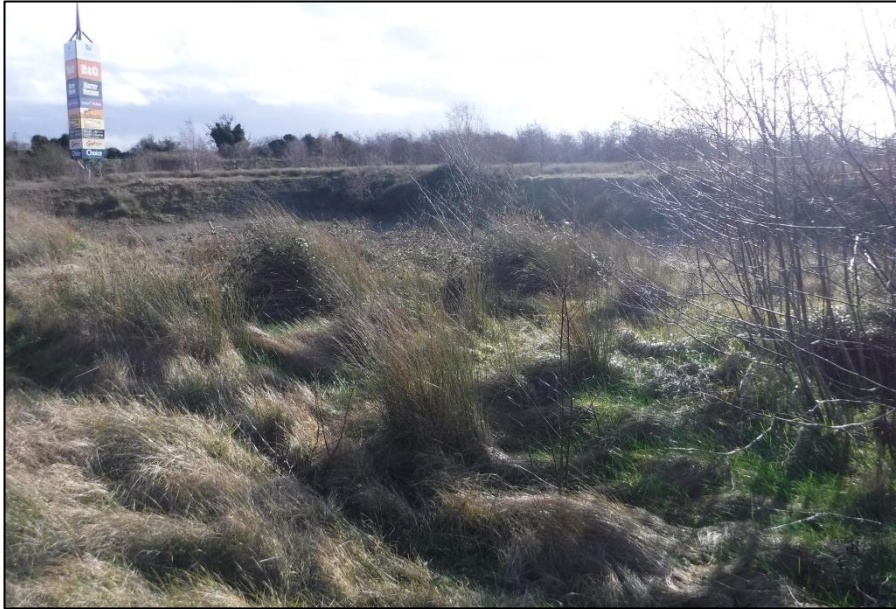
Plate 2 Drainage Features outside eastern site boundary
